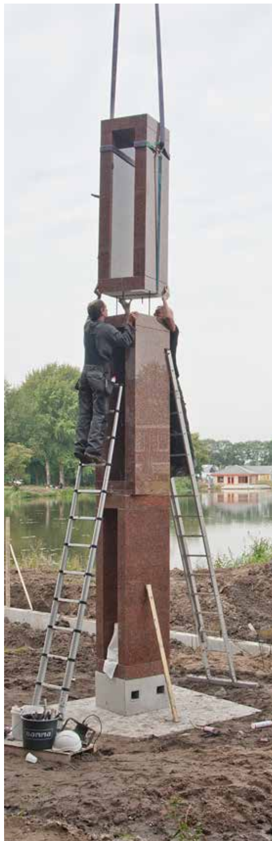
left: 2013, construction of the red granite at Gorinchem, Netherlands sculpture in situ
